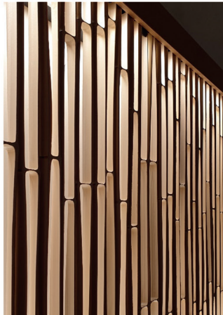
Figures 18, 19. Kengo Kuma, Misonoza, Nagoya, 2017. Cafeteria wall made of bamboo, inside souvenir shop Photographs by Agnese Haijima, 2019
